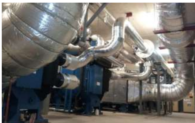
3,516kW Capacity / Gas Engine Exhausted Driven (Australia)
