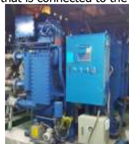
Installation of DWHH100 (2016. 11)
